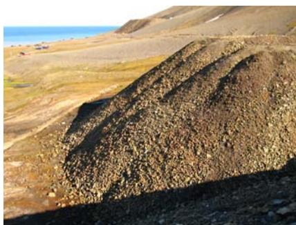
**Figure 1.** The abandoned coal mine waste pile in Bjørndalen near Longyearbyen, Svalbard (78°N). The pile is 20 m high and comprises roughly 200,000 m<sup>3</sup> of pyritic waste rock (<1% FeS<sub>2</sub>) deposited between 1986 and 1996.
